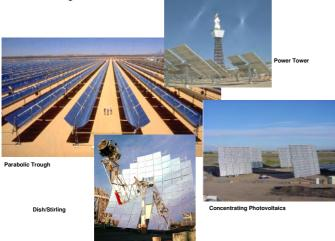
Figure 17. Four different categories of concentrating solar power technologies: power tower, parabolic trough, dish/Stirling, and concentrating PV.
