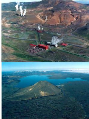
The Háganga hydropower reservoir in the highlands of lceland. Peaking operation of the hydro powerplants support baseload generation from the country's geothermal power stations. The example in the foreground [top] is the 60 MW Krafla plant in northern lceland.
