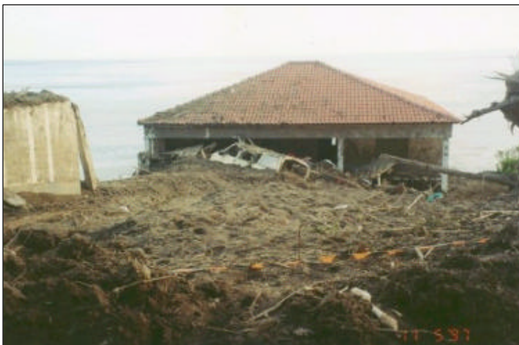
Figure 4.4 House and property destroyed by mudflows in Ribeira Quente
