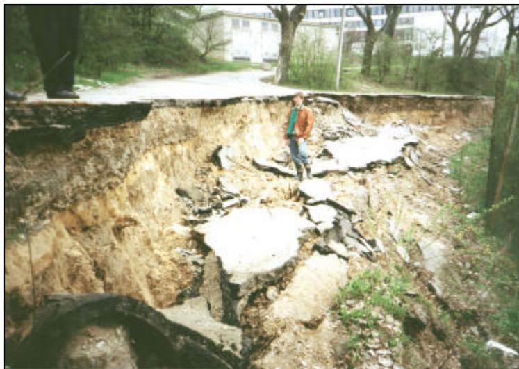
Figure 7.1 Landslide head scarp and destroyed storehouses
