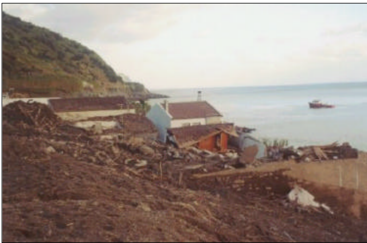
Figure 4.3 Houses destroyed in Ribeira Quente, and mud and debris covering the village
