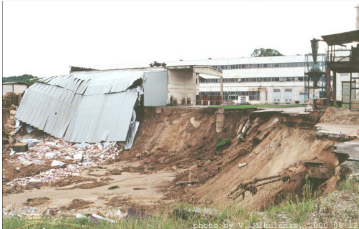
Figure 7.1 Landslide head scarp and destroyed storehouses
