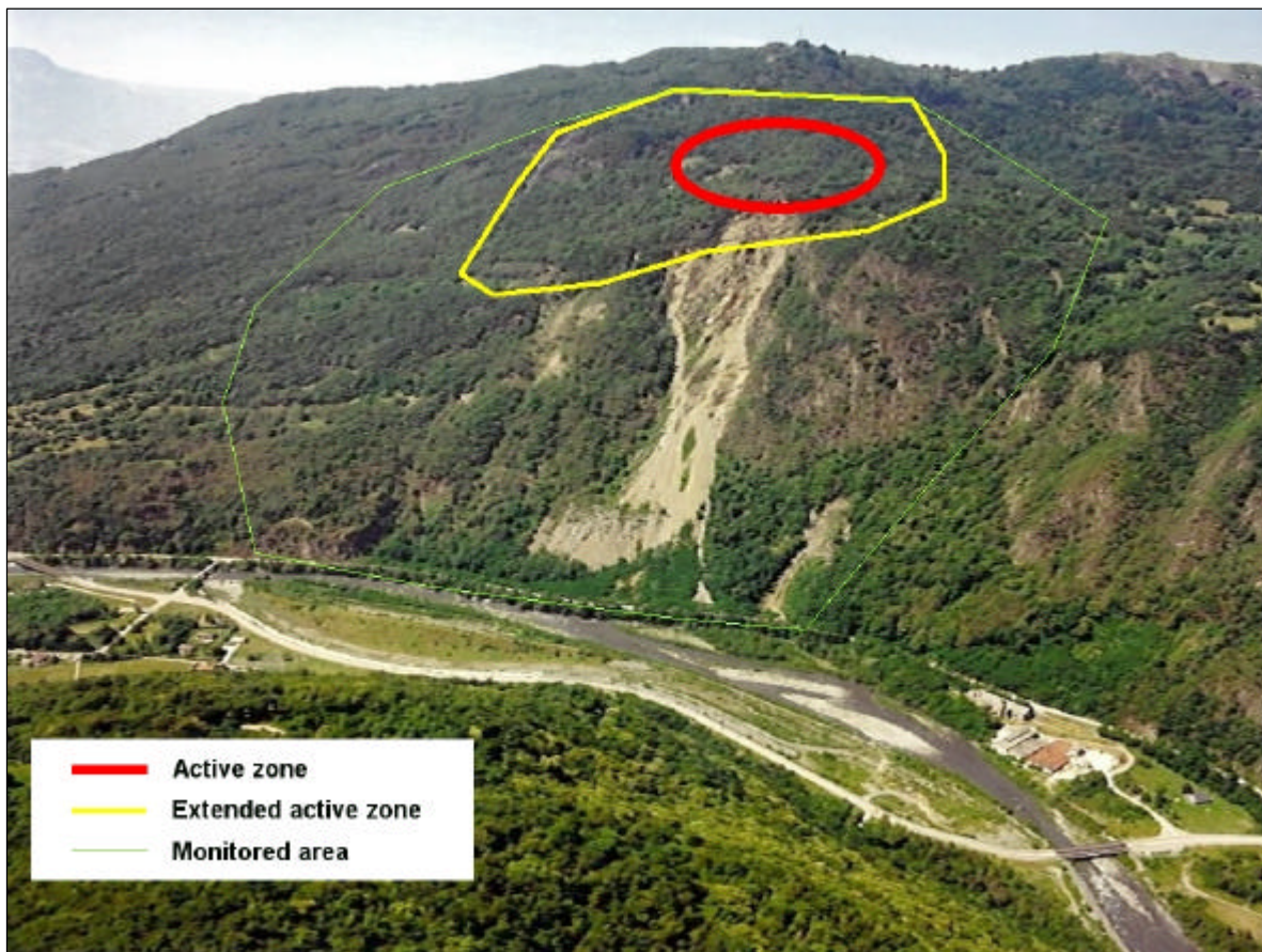
Figure 8.4 Zones considered in future catastrophic mass failure scenarios at Les Ruines de Séchilienne
