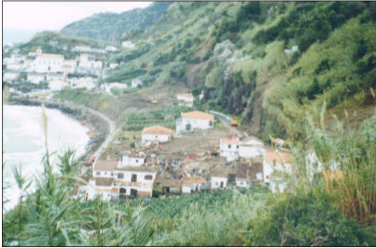
Figure 4.2 Village of Ribeira Quente after the landslides
