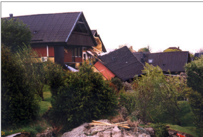
Figure 5.4 House destroyed by the 23 May 1997 landslide
