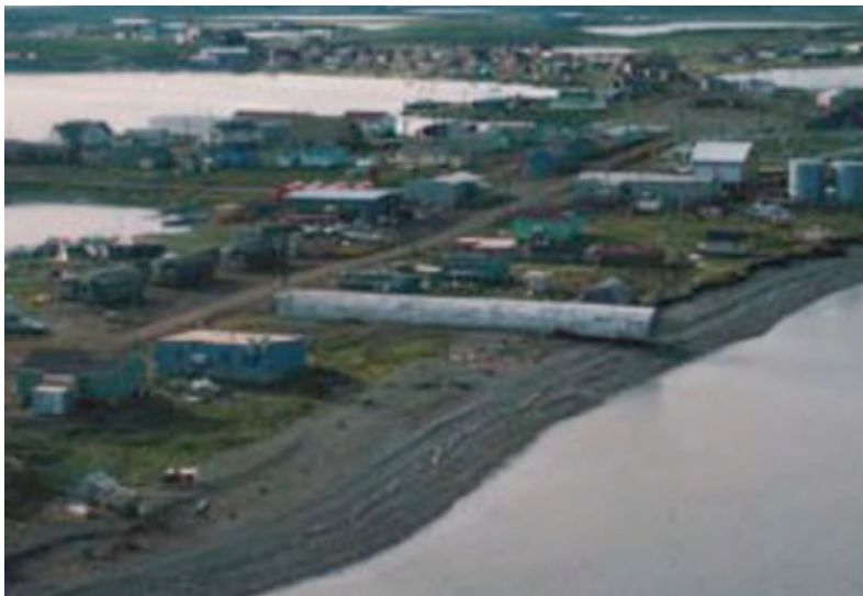
Coastal Erosion in Tuktoyaktuk Photo: PWNHC
