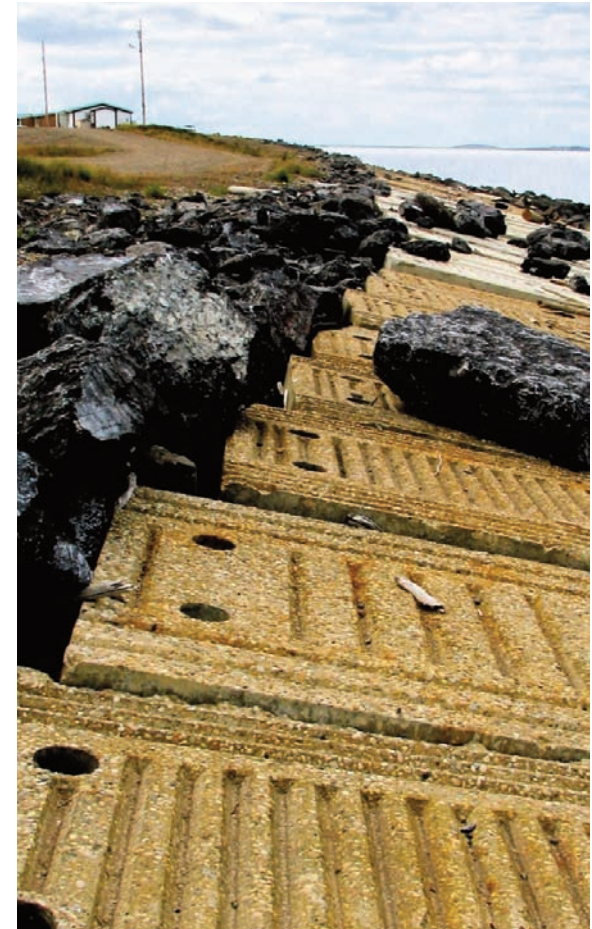
Massive cement barriers piled high on the fragile shores of Tuktoyaktuk where rising seas and more violent storms have cast a shadow over the town's long term future. (Jamie Bastedo)
