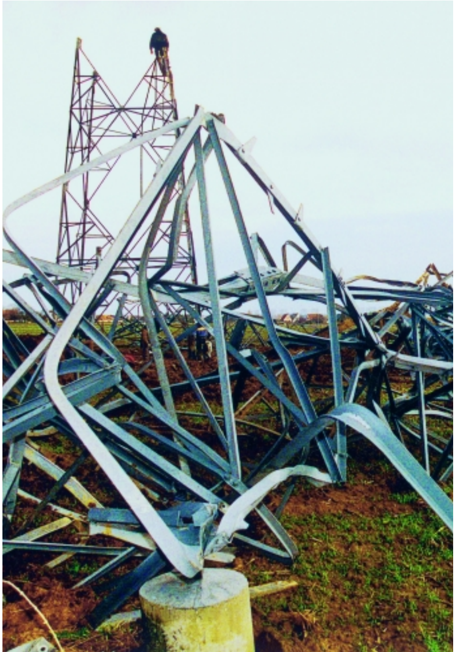
Electricity pylons reduced to scrap metal near Wahlenheim, eastern France.
