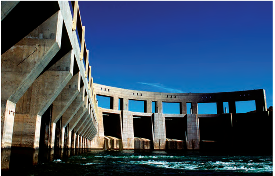
Parker Dam, AZ. Photo courtesy Bureau of Reclamation.
