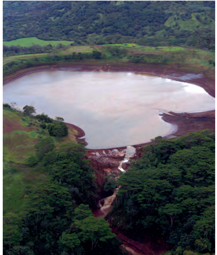
The breach on the 400 million gallon Kaloko Reservoir on Kauai’s North Shore, HI. Image Courtesy of Bruce Asato, The Honolulu Advertiser.
