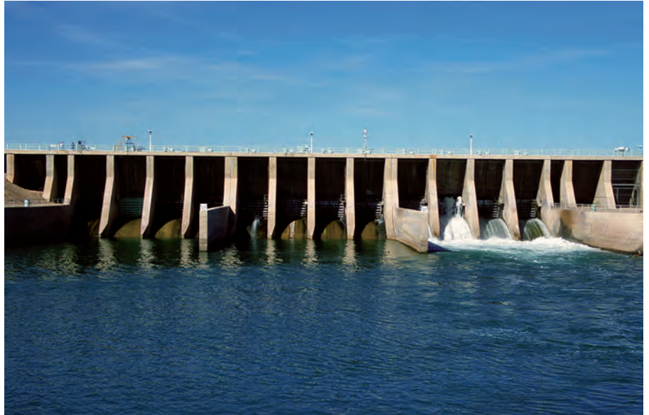
Imperial Dam, AZ. Photo courtesy Bureau of Reclamation.
