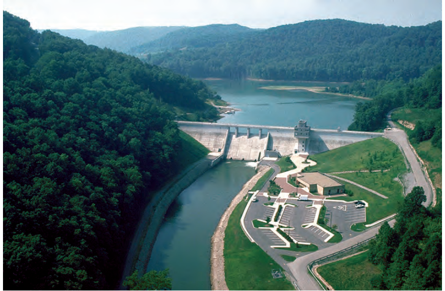
Stonewall Jackson Lake and Dam, WV. Photo courtesy U.S. Army Corps of Engineers.
