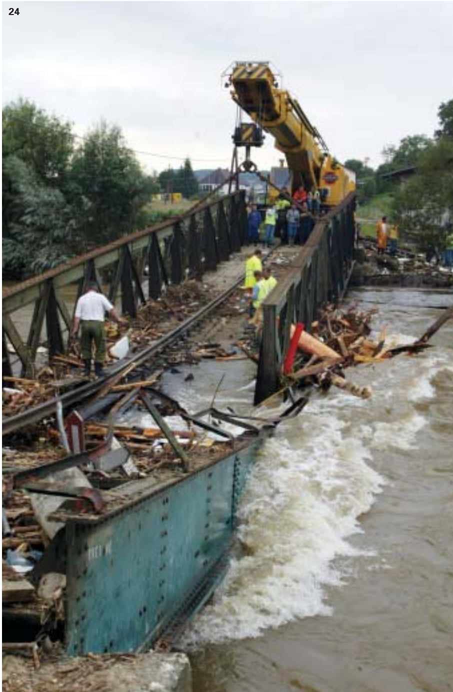
The clogging of bridges with wood and other floating debris is a constant cause of overflows. This is a picture of a railway bridge in Austria which was unable to withstand the forces of the water.
