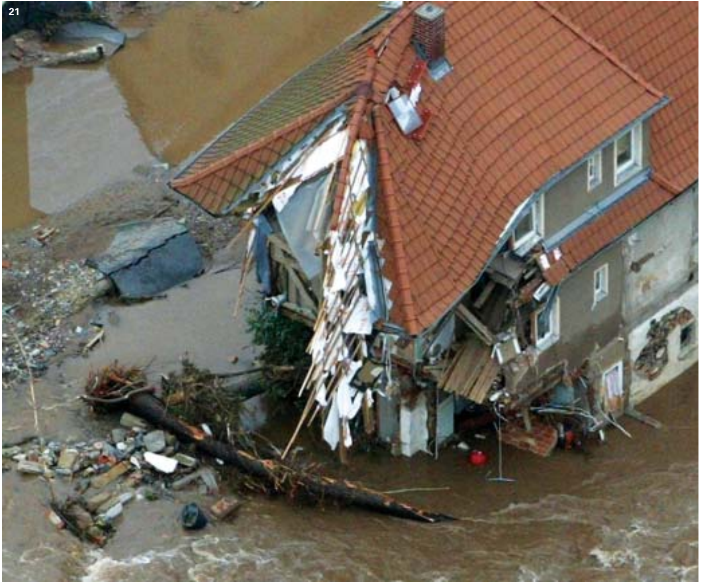
The massive falls of rain at the beginning of August turned small rivers and brooks into raging torrents. Many houses that had been built too near the water were destroyed. The development of areas near rivers is one of the main reasons for the dramatic increase in flood losses in Europe.
