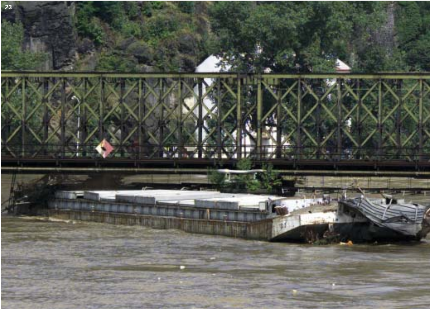
The flood waters on the Vltava were so strong that a number of inland water transport vessels in the Czech Republic had to be blown up with explosives to prevent them from damaging or even destroying bridges.
