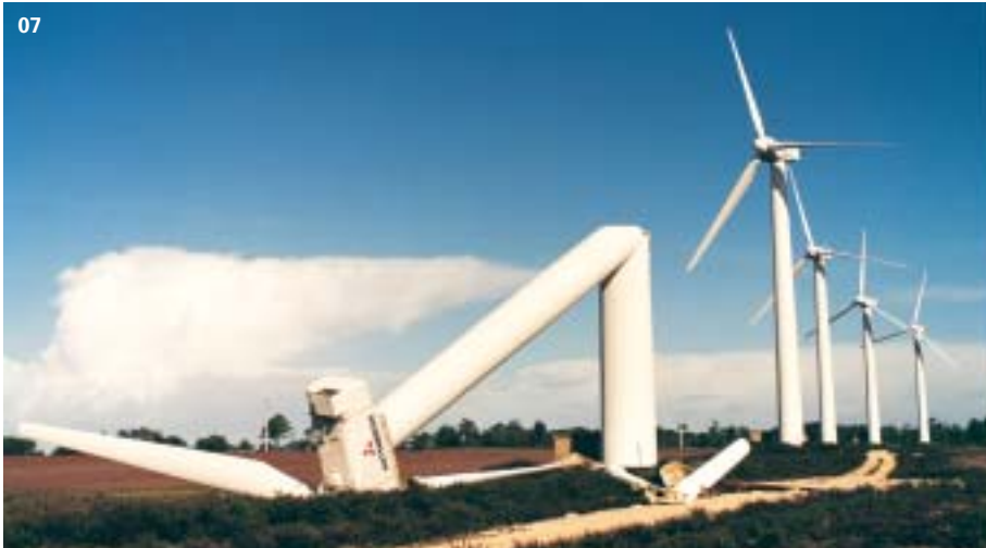
07 The first winter storm of the year, Jeanett, caused enormous damage in many countries of Europe. In Germany, Jeanett could become the costliest insured windstorm loss of all times (insured losses up to US$ 1bn.) This is a wind turbine in northern Germany that was buckled by the storm.
