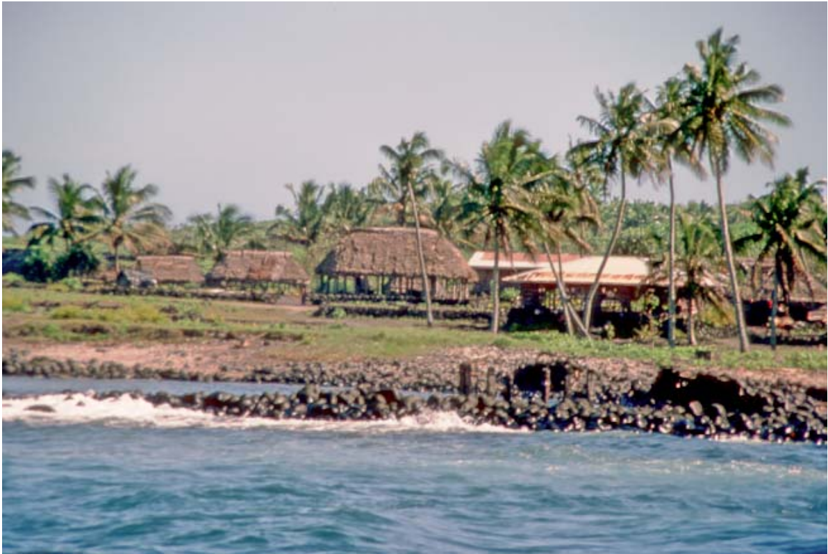
Figure 9 Samoan fale on the island of Savai'i. Note that these buildings have hipped roofs and are placed on significant mounds.
