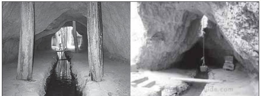
Figure 3. (a) underground canal reinforced with wooden pillars. Source: [www.chinahw.net](http://www.chinahw.net); and (b) outreach of underground canal to surface canal. Source: [www.travelchinaguide.com](http://www.travelchinaguide.com)
