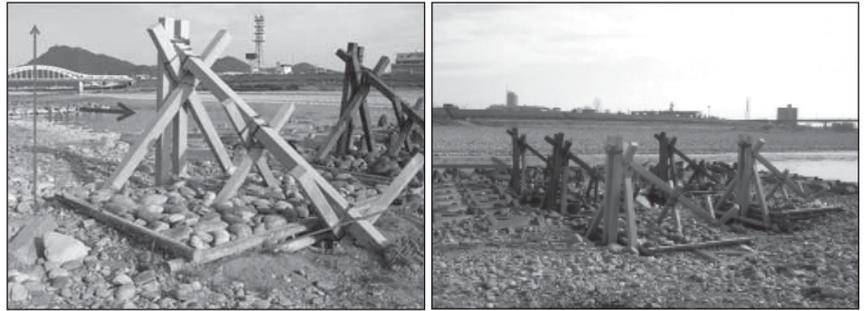
Figure 3. Hijiri-ushi made of concrete (Photo by NIED-KU, 2007)
