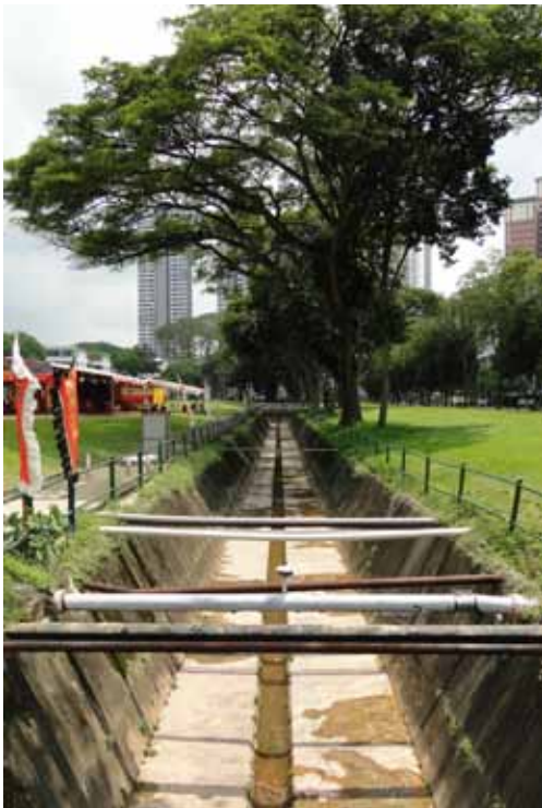
Storm water collection infrastructure is integrated into public green space © UN Habitat/Andrew Rudd
