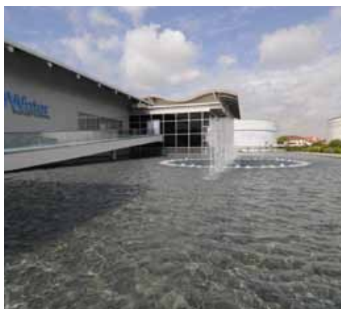
NEWater Visitor Centre, Koh Sek Lim Road, Singapore © PUB, Singapore's national water agency, 2009
