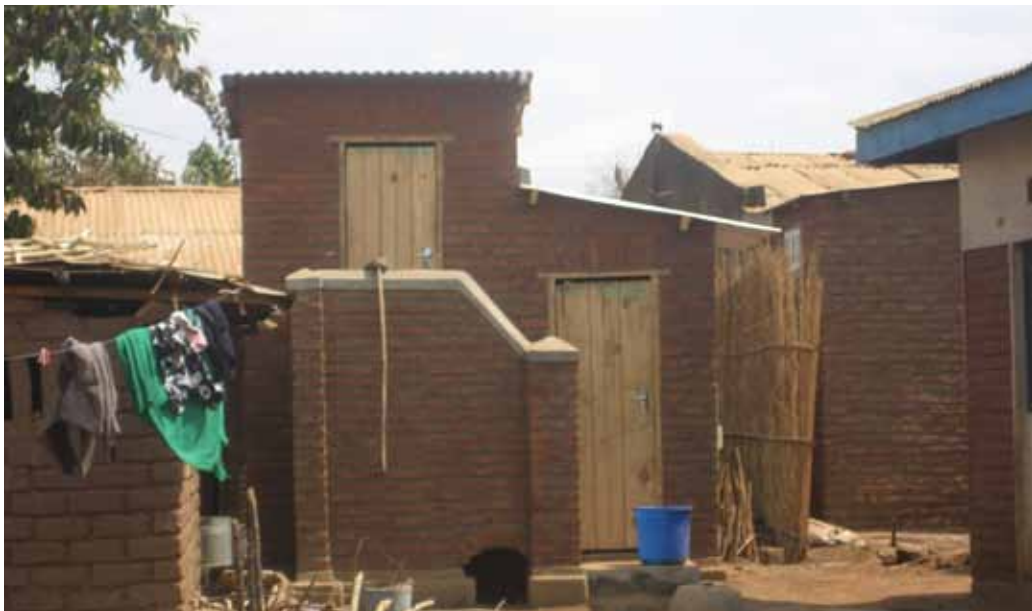
Front view of the ecosan toilet (raised structure on left) and adjoining shower (ground level on right). The ecosan toilet is raised above two composting chambers with access to the chambers at the rear of the structure © Lauren Tavener-Smith, September 2011
