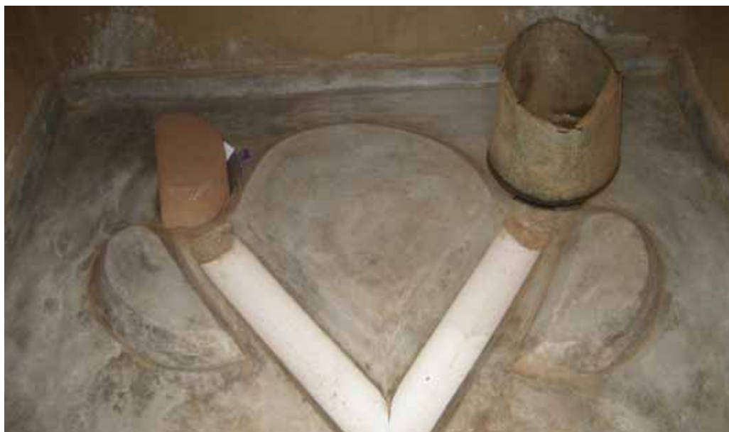
Inside the ecosan squat toilet, urine is diverted through a hole at the apex of the v-shaped gutter where it is soaked away or collected in jerry cans. The brick and bucket cover two holes for faeces, above two chambers. At any one time, one hole and chamber is in use, whilst the contents in the other chamber decompose © Lauren Tavener-Smith, September 2011
