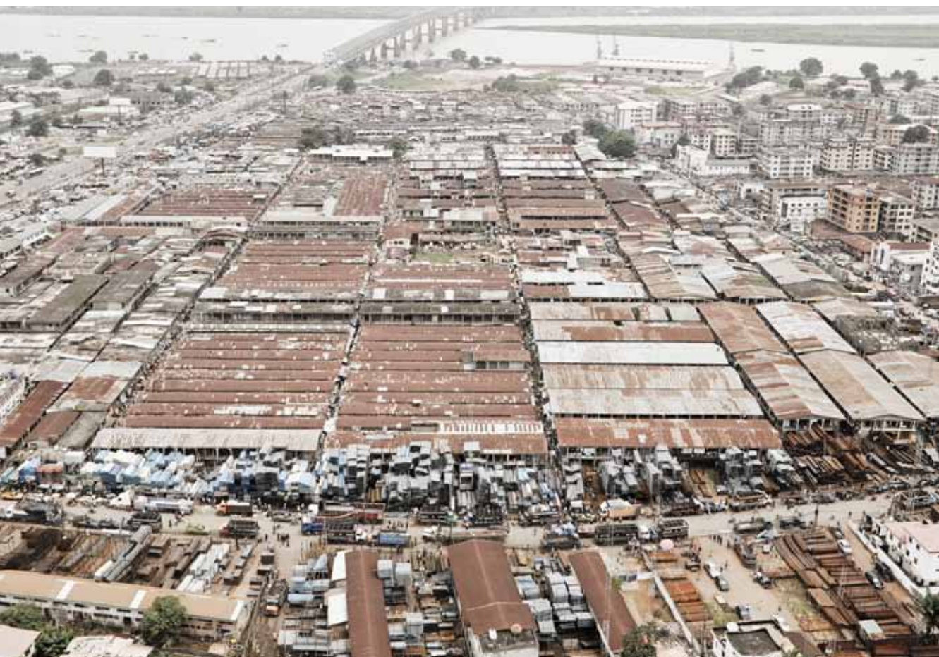
The market area of Onitsha, Anambra State, Nigeria is strategically located at one of the only bridges crossing the Niger River, in this case the Transafrican Highway © UN-Habitat/Alessandro Scotti
