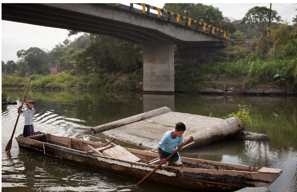
Bridge washed out by flooding and its rebuilt replacement on the Teaone River in Esmeraldas, Ecuador ©UN-Habitat/François Laso
