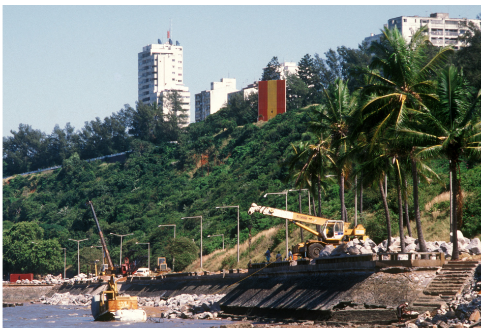
Construction in the coastal area of Maputo, Mozambique ©UN-Habitat/Ricardo Rangel
