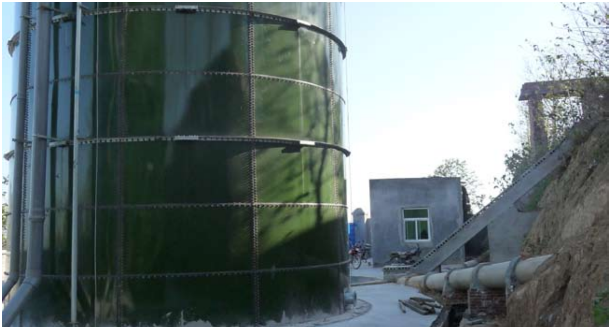
Biogas digester helps reduce emissions and provide clean energy in the PRC, F. Radstake 2008.
