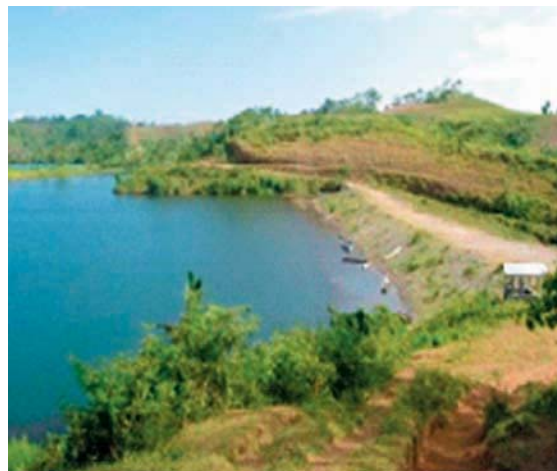
Figure 6.4. Small Water Impounding System in the Philippines
