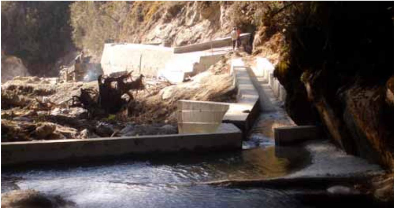
A view of the intake diversion canal. Project: Community Micro-hydro for Sustainable Livelihoods – Sengor, Bhutan.
