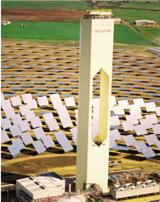
Figure 1: Above, power tower pilot project, pioneered in the U.S. (Barstow, CA) and (left) commercial unit under development by Abengoa called PS10, an 11 MW plant in Sevilla Spain (photo credit: Abengoa Solar). Bottom left, Stirling Dish/Engine, Center SEGS trough plants, Right, Compact Linear Fresnel Reflector.
