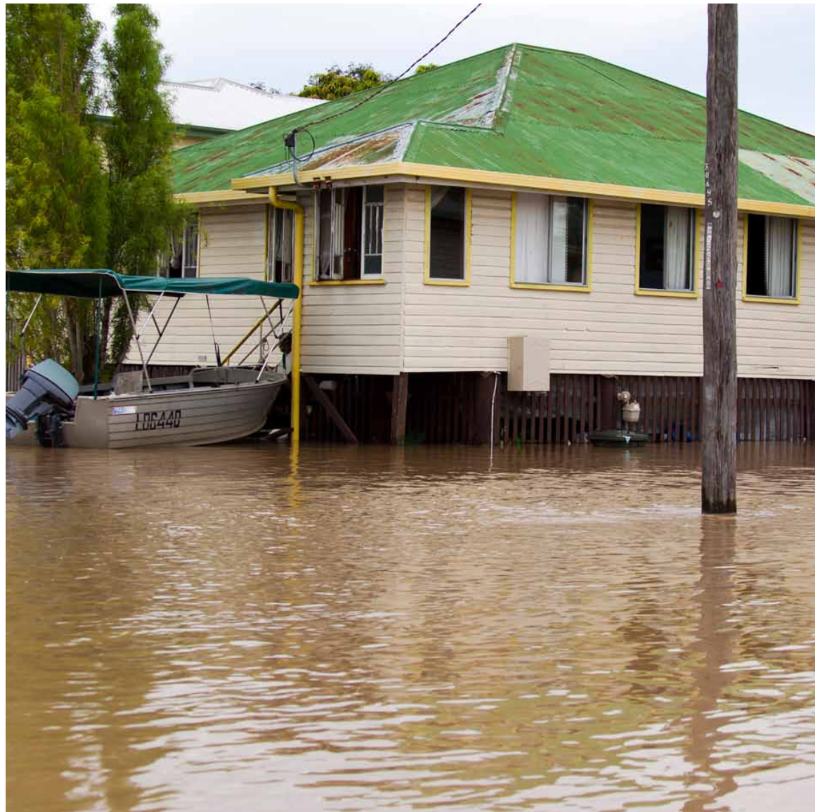
Photo: In flood prone areas, houses with habitable floors built above the potential flood height can reduce the loss and damage associated with floods. Photographer: Michael Marston
