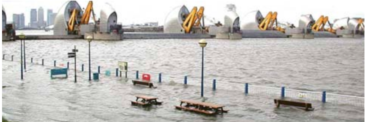
Surge tide event at the Thames Barrier
