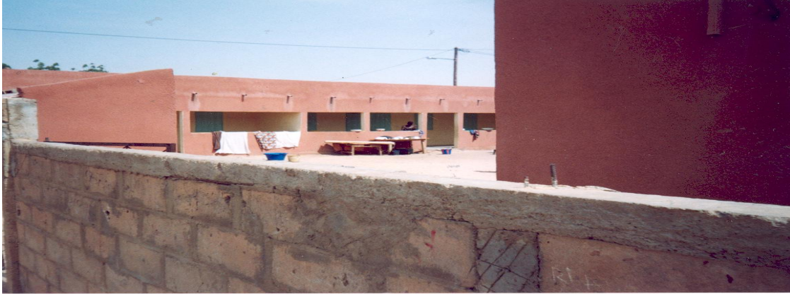
Photo 1: Construction of individual rental apartments
