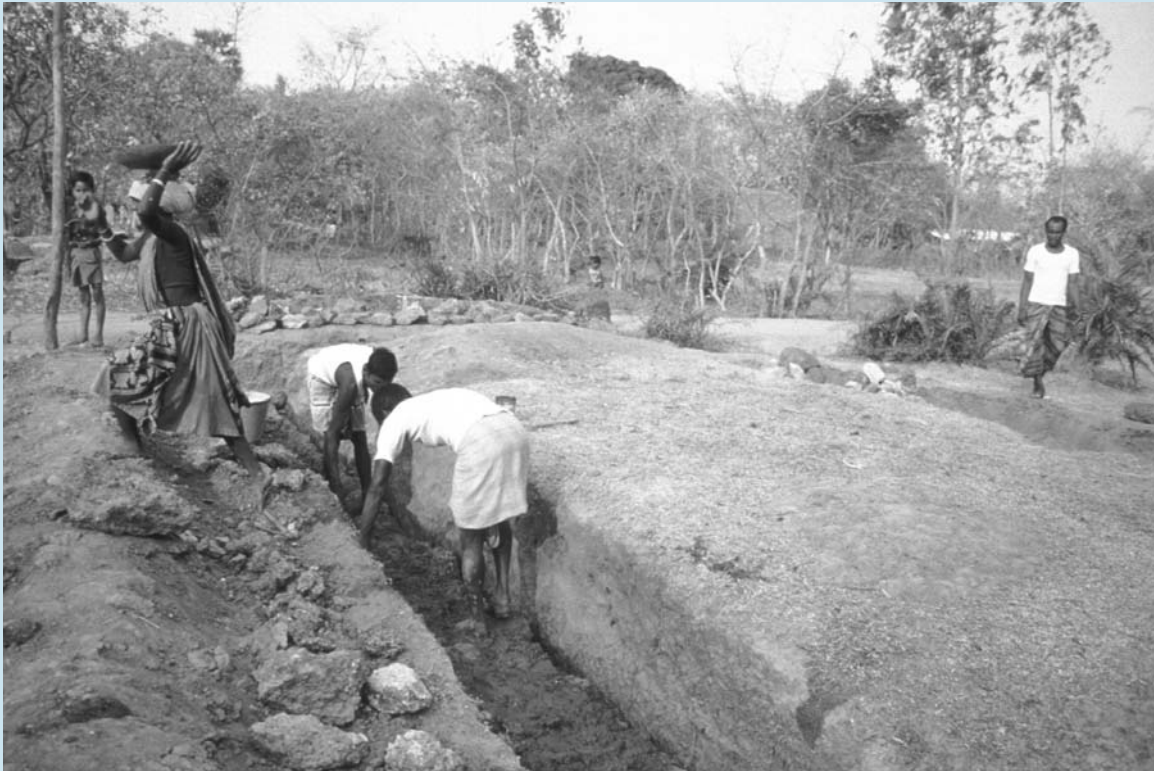
Workers digging irrigation ditch in India. Photo by Curt Carnemark, courtesy of World Bank Photo Library.
