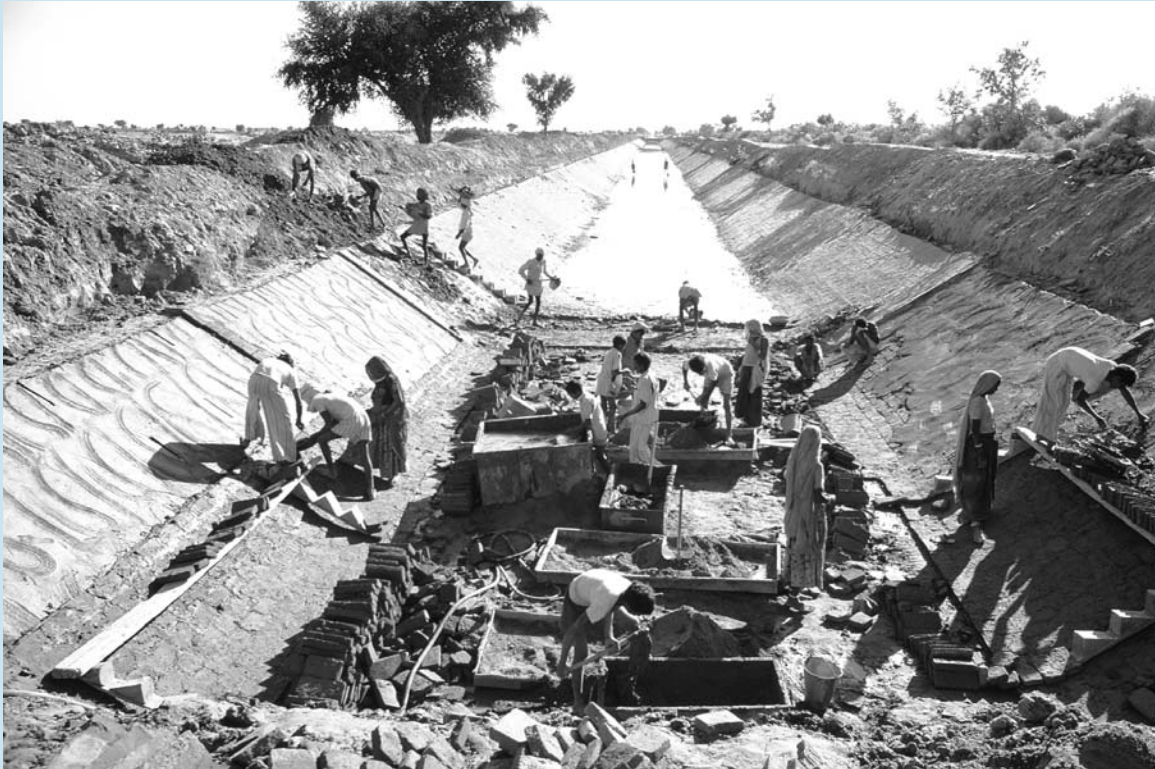
Building a brick main canal in India. Photo by Curt Carnemark, courtesy of World Bank Photo Library.
