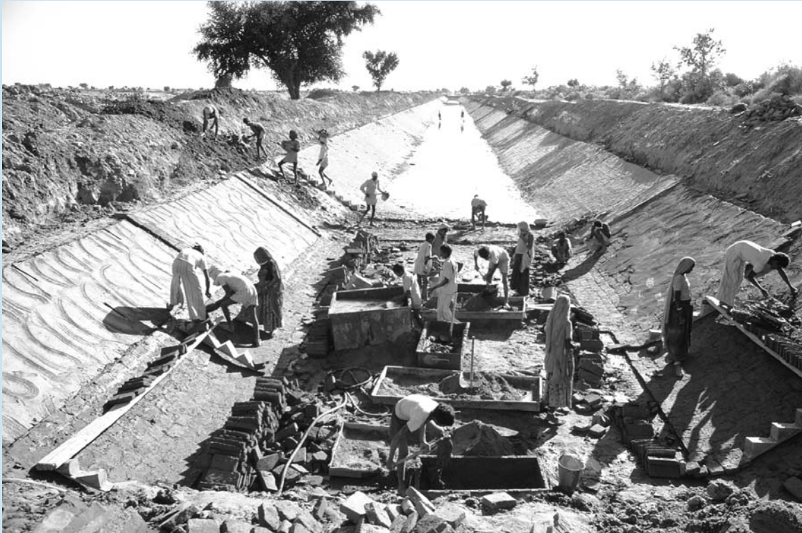
Building a main brick canal in India. Photo by Curt Carnemark, courtesy of World Bank Photo Library.
