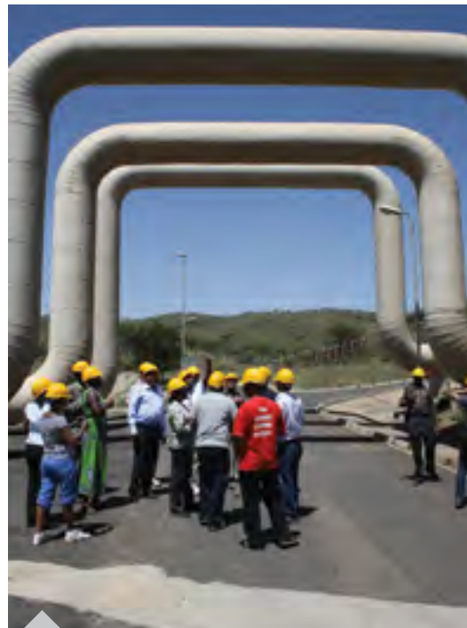
A field trip to Kenya's Olkaria geothermal power plant during the March 2012 SREP pilot countries meeting offered a first-hand look at the technology and sparked discussion. Photo: CIF
