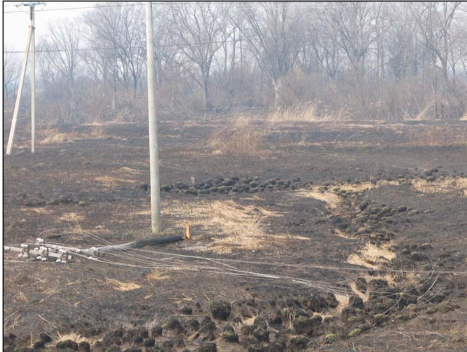
Figure 23. Infrastructural damages caused by the 2010 wildfires in Western Russia are not yet accounted. ©Photo: GFMC.
