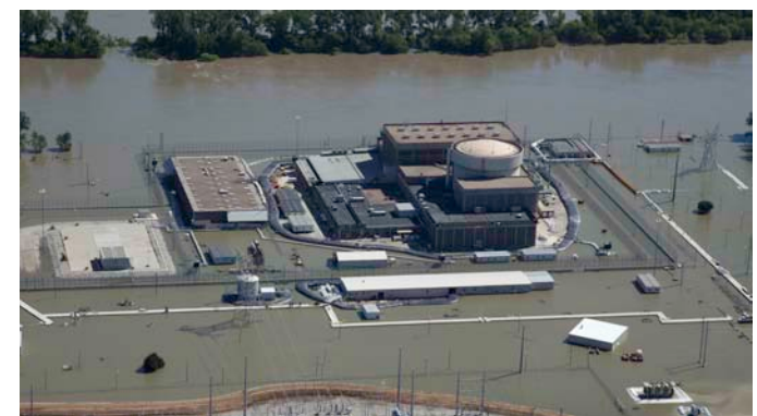
Figure 27. Flooding of the Ft. Calhoun nuclear power plant in Nebraska, spring 2011
