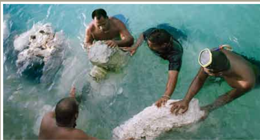
Pieces of coral removed from the reef are used to form a wall to help protect the foundations of a church building in Kiribati, Tarawa
